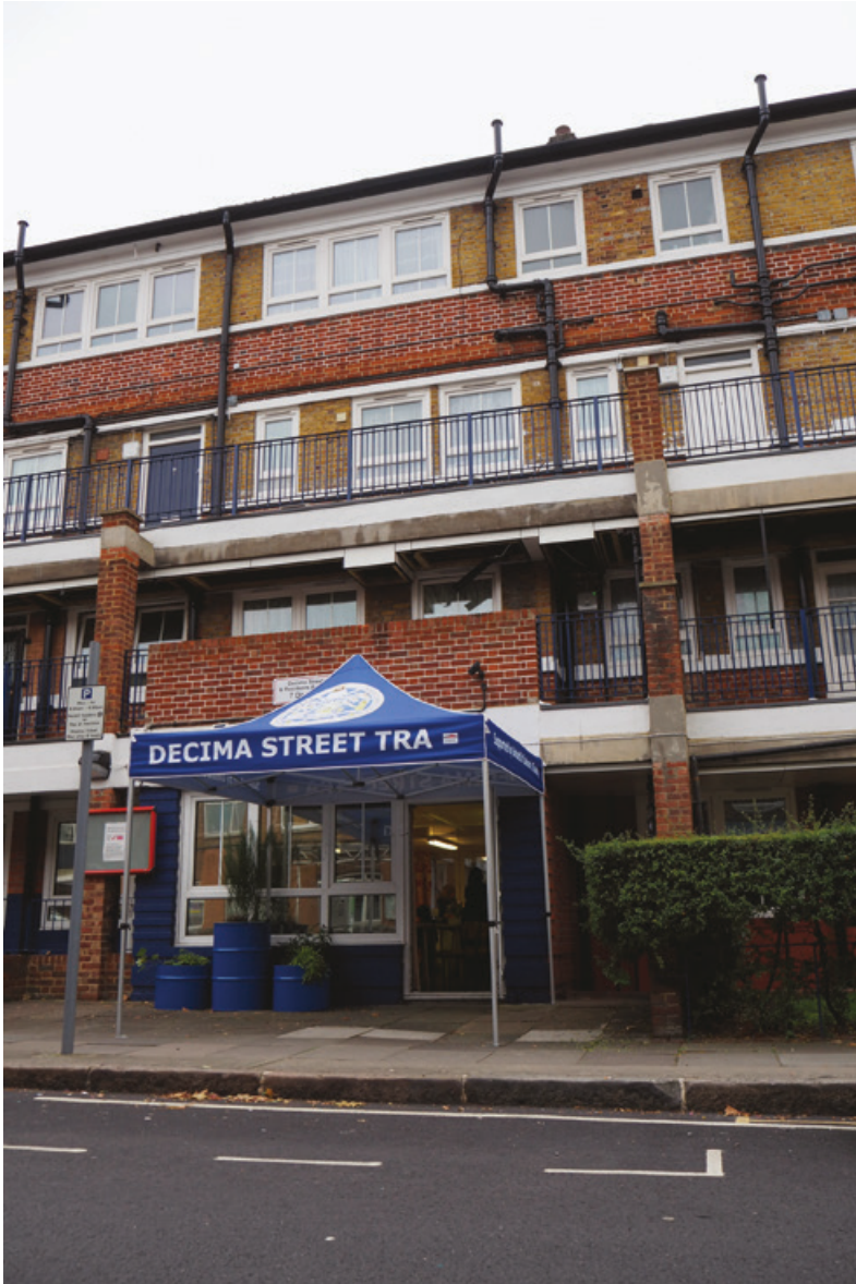
Figure 6.3 View of Meakin Estate and the TRA meeting room from Decima Street
